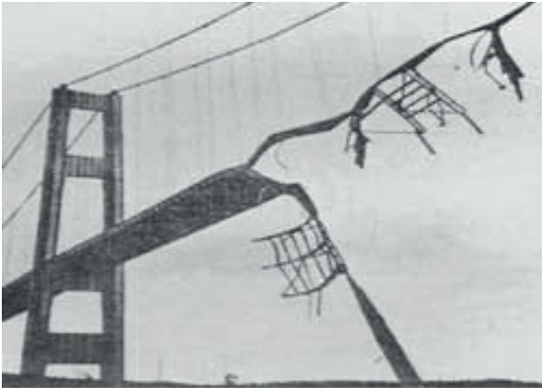
Fig. 3 Instorting van de Tacoma Narrows Bridge door flutter
